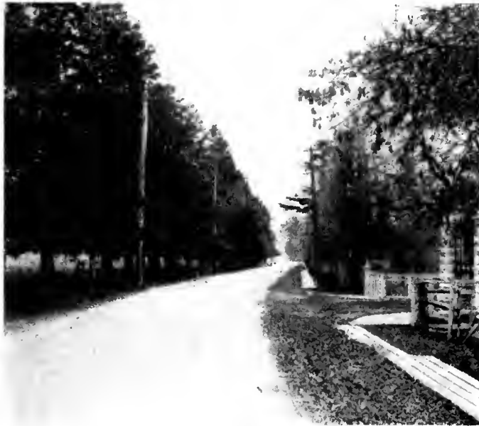
Montreal-Quebec Road at Ste. Foy. Asphaltic concrete surface laid in 1917 by Quebec Department of Roads.
